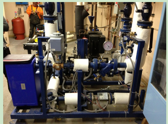
HHW heat exchanger skid installed at Sweet Hall in place of old steam heat exchanger
